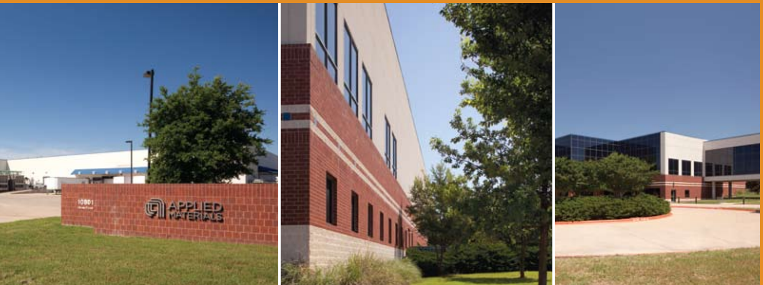
Left to Right: Loading entry signage. Building 36 exterior. Building 30 entrance
